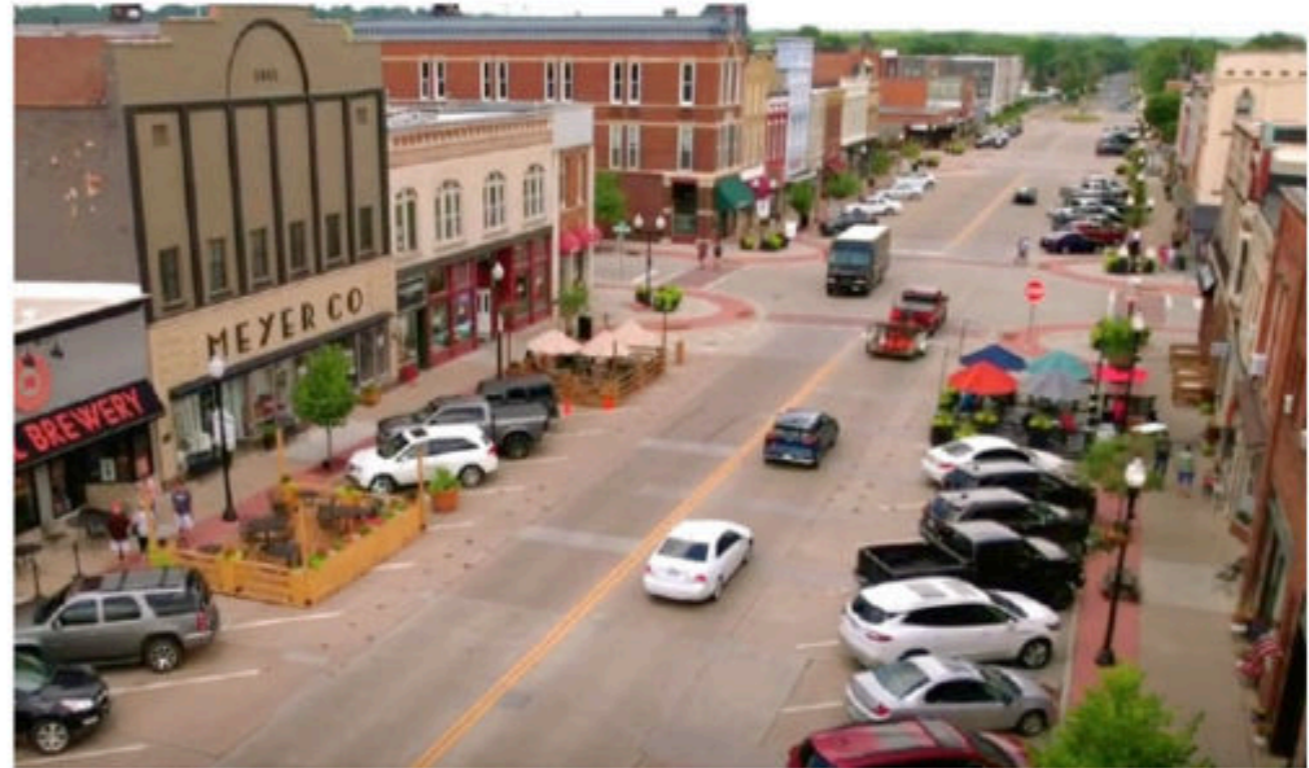
New parklets, outdoor seating, and streetscape in Hastings MN.
